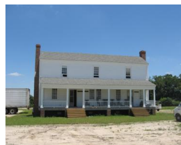
“Cederville” moved, painted and full of workers. Looks great!
